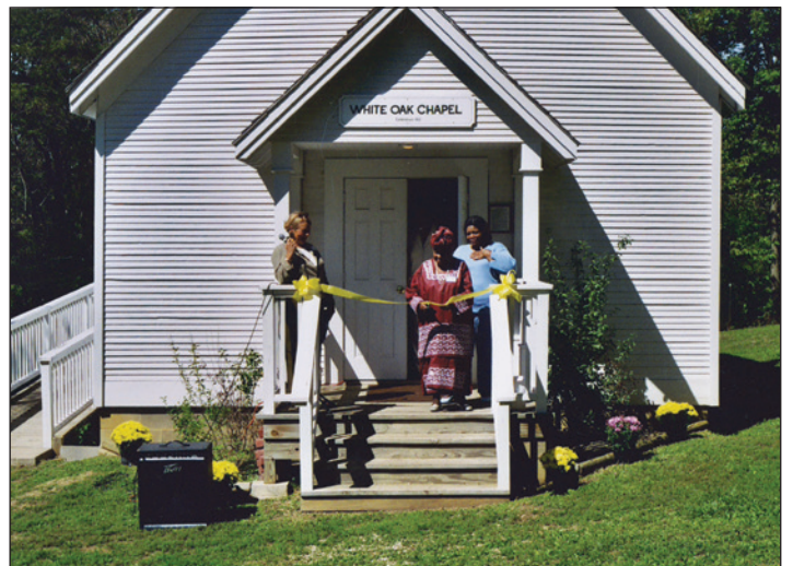
A descendant of an original member of the congregation cuts the ribbon at the White Oak Chapel ceremony. As the Friends of Sacred Structures's first large-scale relocation project, it is the best-documented collaboration in the collection.
