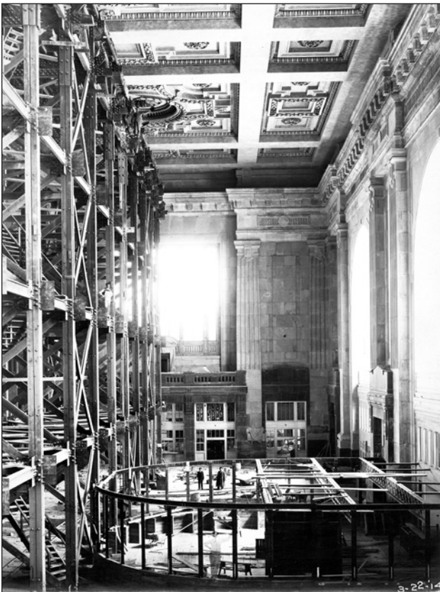
Taken on March 22, 1914, this photo shows construction of the Grand Lobby in Kansas City's Union Station. Work on the building, designed by Jarvis Hunt, a proponent of the City Beautiful Movement, began in 1911.
