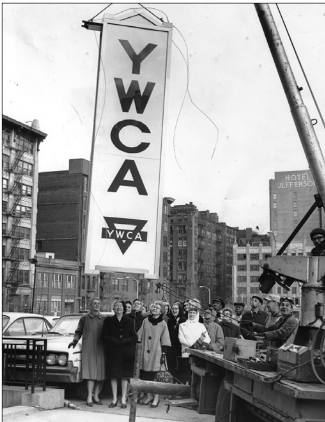
Installing the YWCA Central Branch sign at 1411 Locust Street in St. Louis, 1964. The YWCA of Metropolitan St. Louis was founded in 1904.
